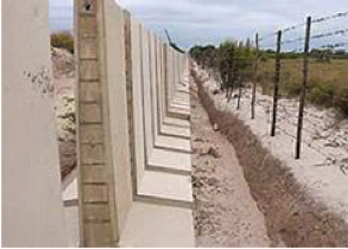
Now the wall is...
