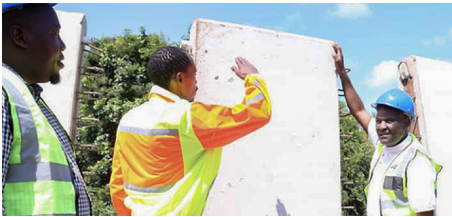
Workers at the wall
