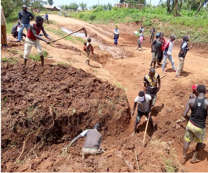
Arranging access roads to the camp
