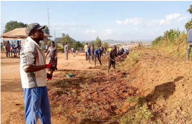
Preparing the ground for shelters
