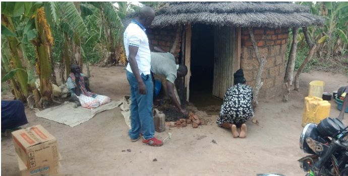
Repairing an old lady's house
